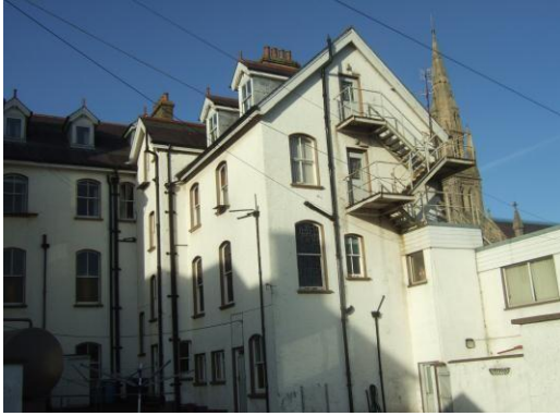
Building to the far-right is now the CCMS Office
